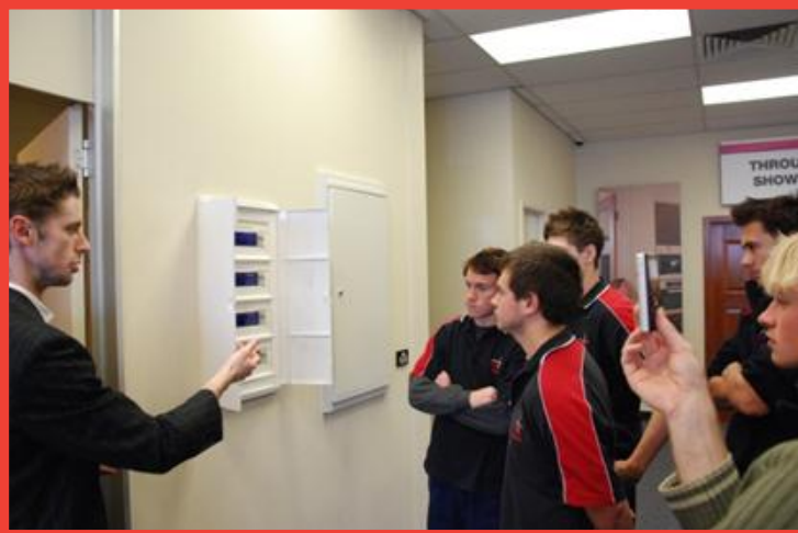
Above: The students viewing the control centre of the Home Automated System
